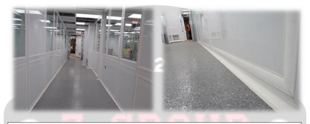
Second Phase of GMP Cleanroom System using Universal Coving System at all wall-to-wall, wall-to-floor, wall-to-ceiling, and all inside 90° corners. The soft edge forms tight against all surfaces to produce an easy to clean radius. Inside corner junctions use a single piece 3-way inside corner.
