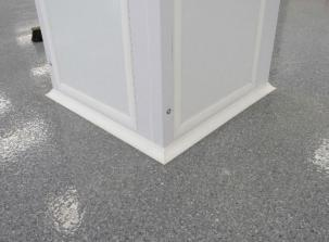
This GMP Cleanroom System used our Universal Coving System at all wall-to-wall, wall-to-floor, wall-to-ceiling, and all inside 90° corners. The soft edge forms tight against all surfaces to produce an easy to clean radius. Inside corner junctions use a single piece 3-way inside corner.
